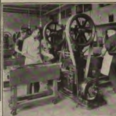
2. The strips being passed through a machine which cuts out disks.
